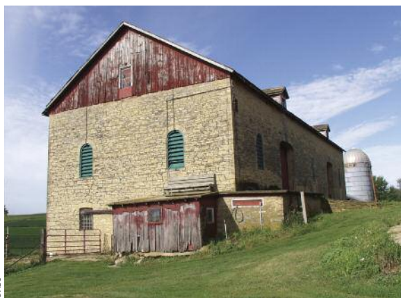
The Thomas Barn, view from the east
